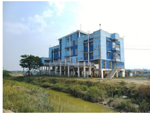
Fig: Cyclone Shelter
