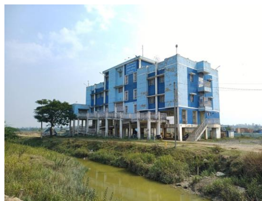
Fig: Multipurpose Cyclone Shelter
